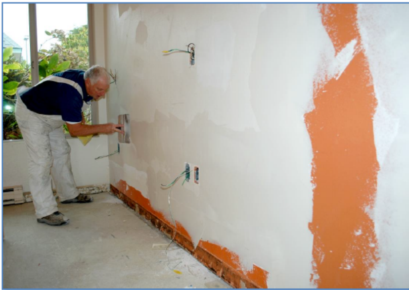
In photo, Lance Boyce muds one of the HPEC rooms.
