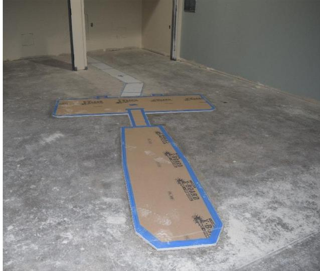
Above, in the CT room in Imaging, a floor leveling epoxy (under the cardboard) has been installed to hold the CT scanner; below, in the main entrance, framing is being done for the fireplace, adjacent to the stairway
