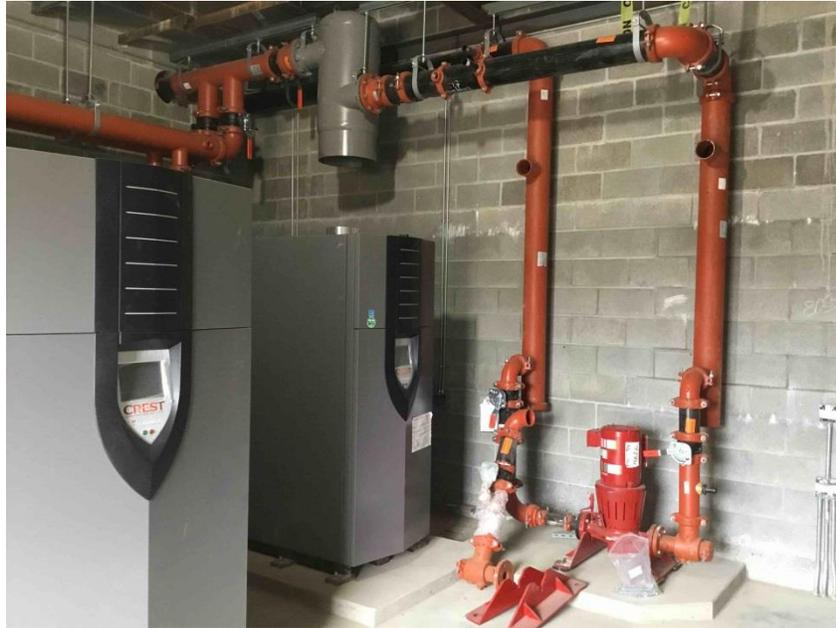
*New hot water condensing boilers are already in place.
