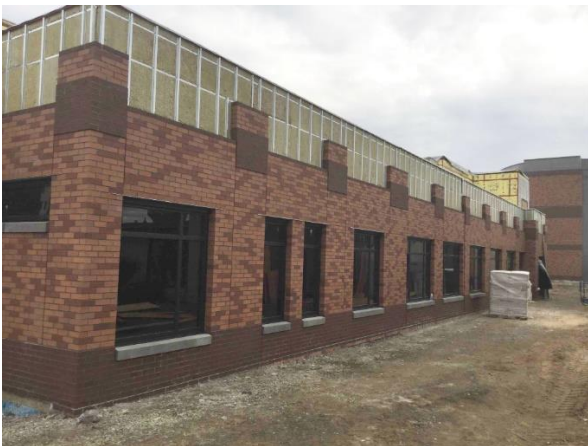
West side brick work is complete
