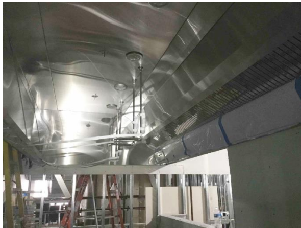
Shiny new kitchen hood has been installed
