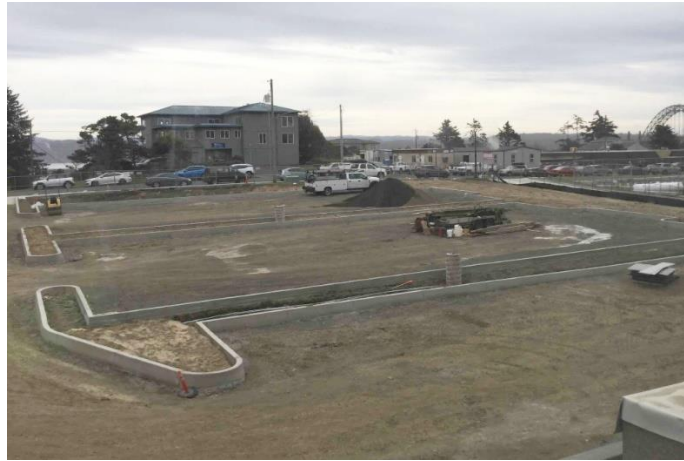
East parking lot site grading and utility installation in-process
