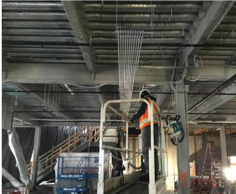
*Inside, this guy is installing fire sprinklers. Look closely and you can see the fireproofing paper mache-like materials clinging to beams. Neenan Co. photo*
